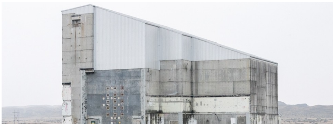
Fig. 5: C-Reactor in the entombed, cocooned state still standing today at the Hanford Site, Washington
