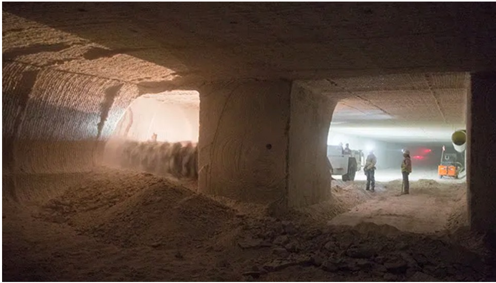
Fig. 3: The interior space of the geological repository during its construction phase
