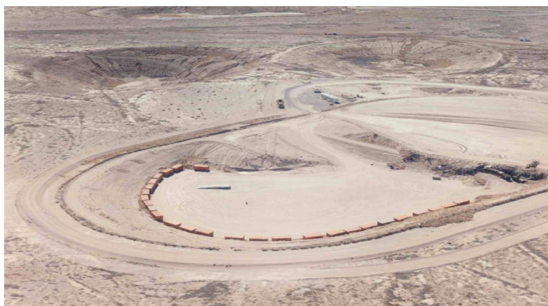
Fig. 4: Area 3 of the Radioactive Waste Management Site, constructed within multiple craters
