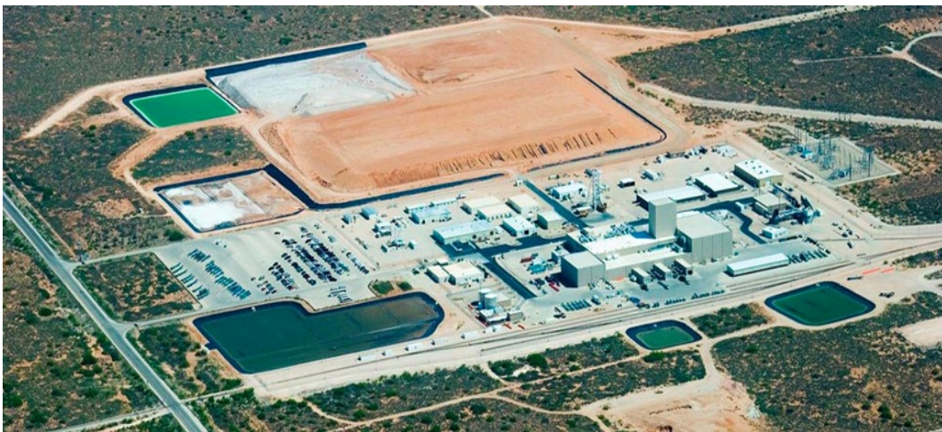
Fig. 1: An aerial view of the Waste Isolation Pilot Plant
